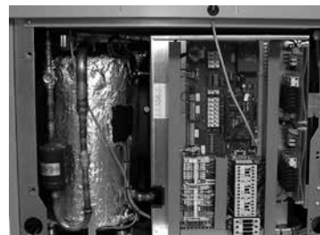
Example of open electrical switch cabinet...
